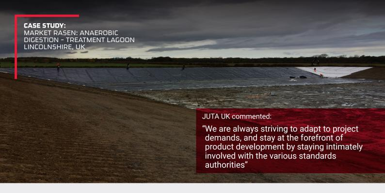
The treatment lagoon at Market Rasen is formed by the creation of an earthworks bunded area, which is then lined with JUTAMAT 5000 (GCL) as a secondary containment liner; overlain by JUNIFOL HDPE 2.0 mm geomembrane as the primary containment liner.
