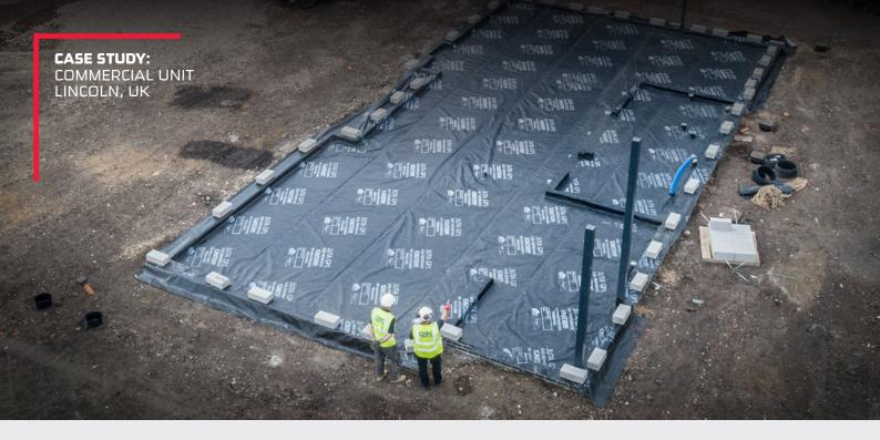
Preparation is key when installing proprietary gas membrane, to both avoid damage occurring during the installation and avoid delays when independent verifiers check the installation according to CIRIA C735. JUTA UK recommend Automatic Twinny Welders to specialist installers to ensure a quick and easy installation. The scheme was installed by specialist installers to NVQ2 with heat welded joints to provide a robust solution to provide a future proof solution for the lifetime of the building.
