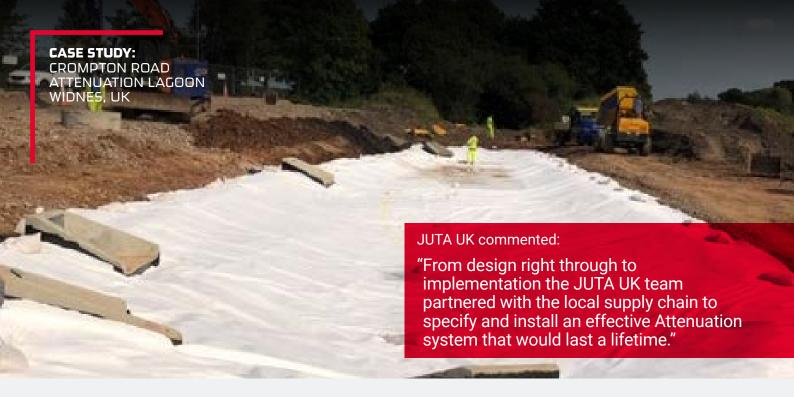
Attenuation lagoons help to control stormwater runoff and are considered the most effective temporary method for storing excess water on site.
