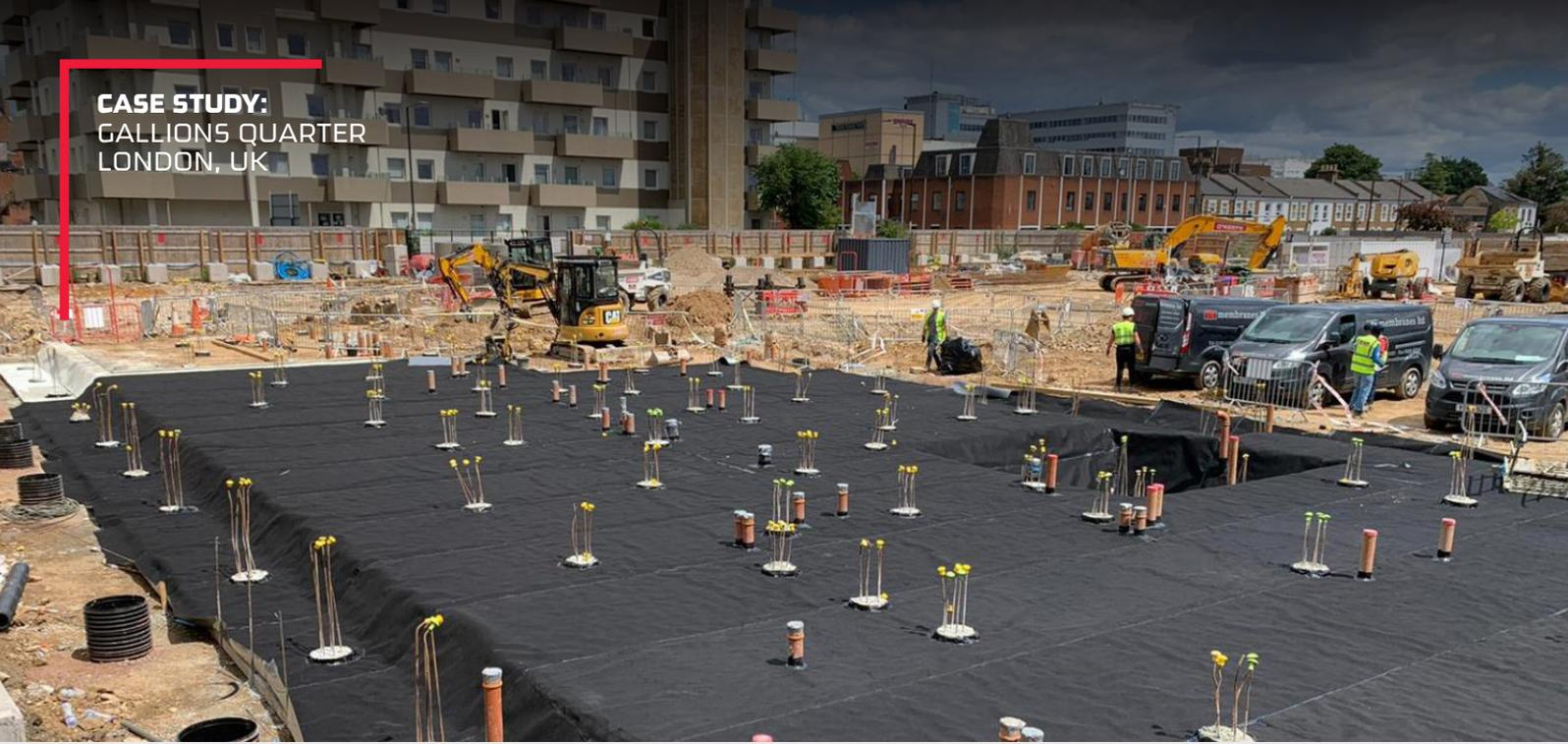
GP® TITANTECH® membranes are the first products of their kind to combine water resistance with protection against hazardous gases, VOC vapours, hydrocarbons and other chemicals that may be present in contaminated land; providing an innovative and durable solution to problems faced with many development sites across the globe.
