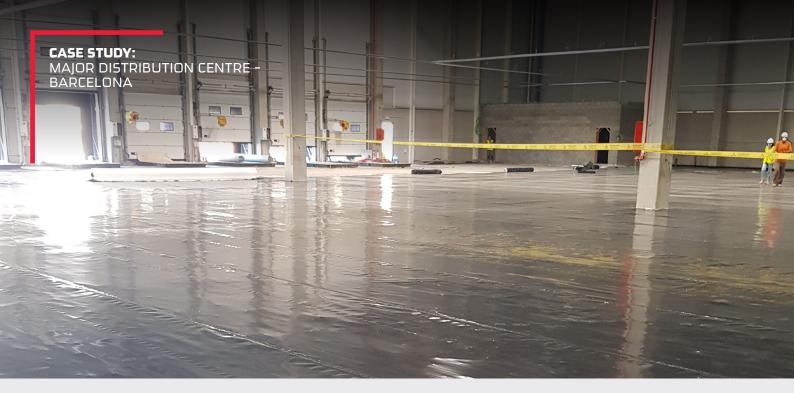
Acciona Construcción approached JUTA UK early 2021 to help with the design, supply and install of 25,000 m² gas protection for a high profile site with a partial basement construction. The previous site use, situated close to the railway line had left residual hydrocarbon contaminants in the ground, and commonly used geomembrane materials were not able to provide sufficient protection.
