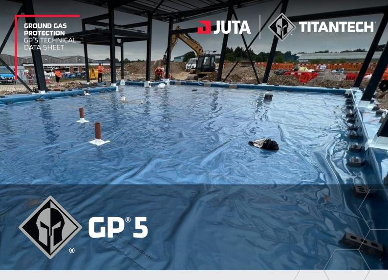
GP®5 gas barrier is a multi-layer composite of virgin polyethylene (PE) giving exceptional resistance to the passage of ground gas and organic vapours. It also acts as a high performance DPM.
