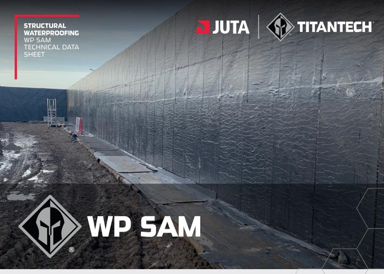
WP SAM - waterproof self adhesive membrane, is a bituminous water proof sheet, composed of self adhesive SBS polymer modified bitumen with an upper surface finish of grey co-extruded polyolefin, and a lower surface finish of siliconized release paper. WP SAM is used for the waterproofing of underground structures, and to prevent the ingress of radon.
