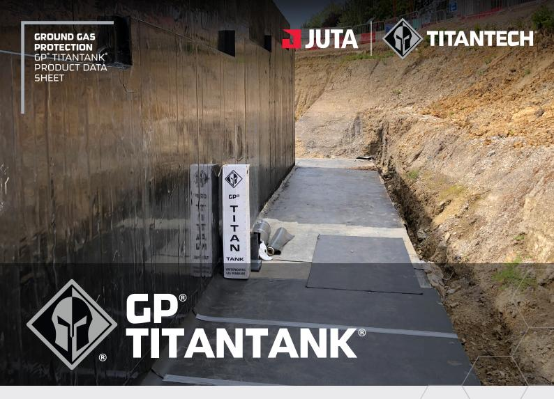
GP®TITANTANK® is a self adhesive version of the GP®TITANFLEX® with an upper surface finish of GP®TITANFLEX®, and a lower surface finish of siliconized polypropylene release film.
