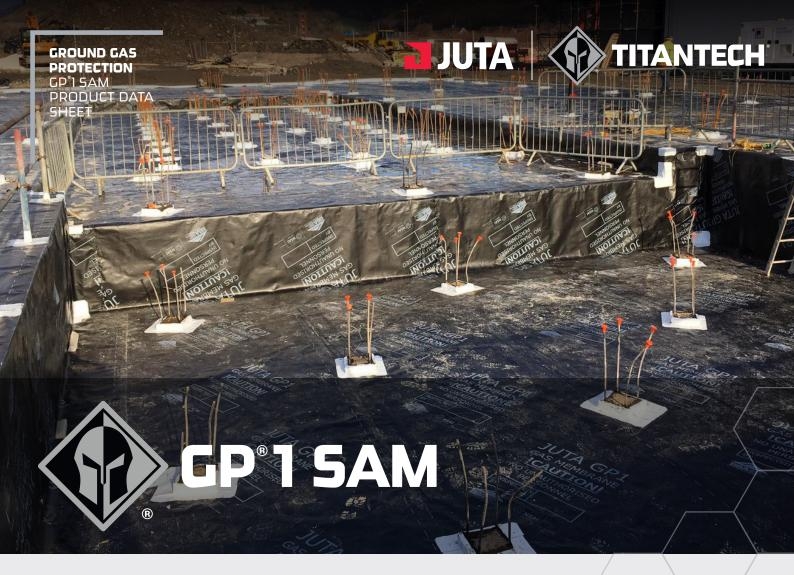
GP®1 SAM, the gas protection self adhesive membrane, is a bituminous gas proof and water proof sheet, composed of self-adhesive SBS polymer modified bitumen incorporating GP®1 with an upper surface finish of black reinforced LDPE, and a lower surface finish of siliconized release film.
