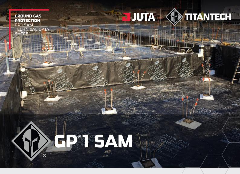
GP®1 SAM, gas protection self adhesive membrane, is a bituminous gas proof and water proof sheet, composed of self-adhesive SBS polymer modified bitumen incorporating GP®1 with an upper surface finish of black reinforced LDPE, and a lower surface finish of siliconized release film. GP®1 SAM is used for the gas/waterproofing of underground structures where harmful ground gasses are anticipated, and as a self adhesive accessory to GP®1.
