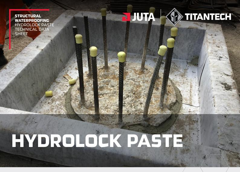
HYDROLOCK PASTE is a plastic bentonite paste which is specifically designed for structural waterproofing. HYDROLOCK PASTE is very easy to use, has excellent water absorption capacity and is biologically harmless, weather resistant, solvent free and frost resistant.
